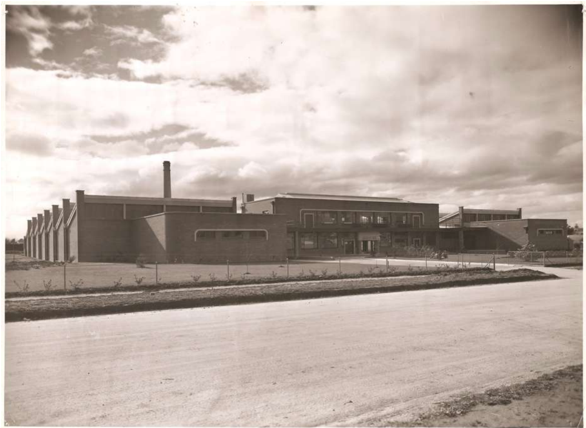
Figure 2: Millers Factory c.1948. Photographer: Doug McClelland. Source: Warragul & District Historical Society
